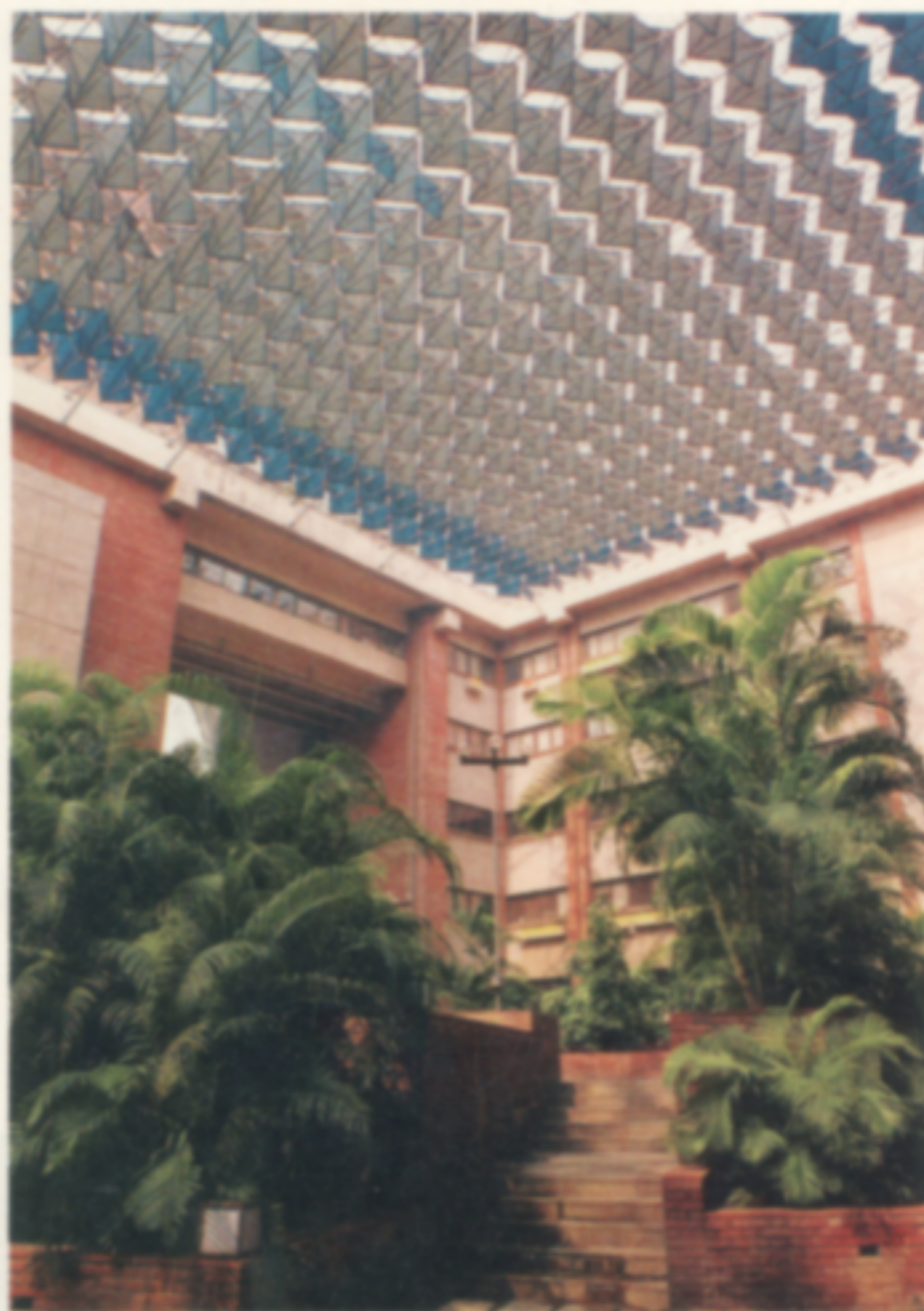
Thirty years later, at the India Habitat Centre (right), Stein shaded courtyards with adjustable webs of louvers, making these acre-wide spaces surprisingly cool and intimate.
